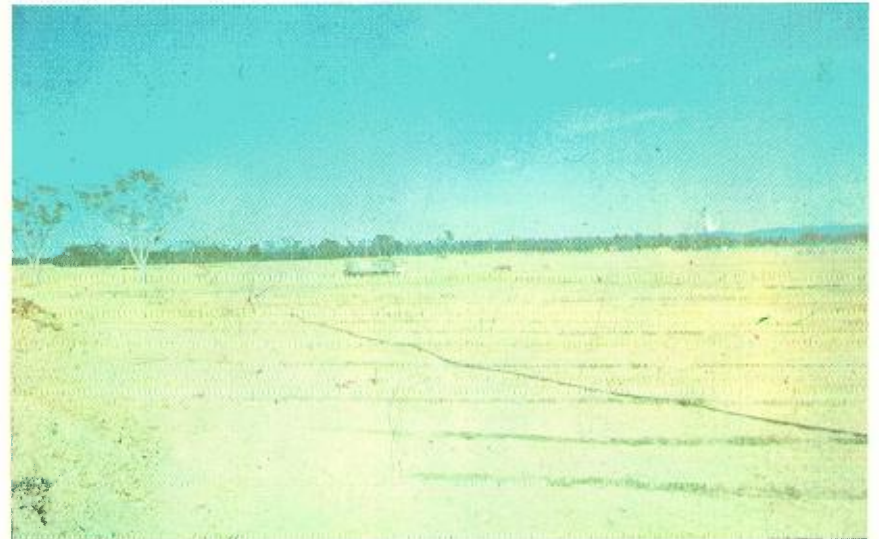
Commencement of restoration operations after final grading of working areas
