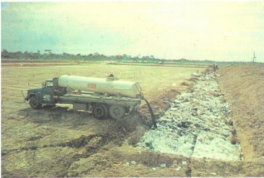
Liquid waste being deposited into cells filled with solid waste
