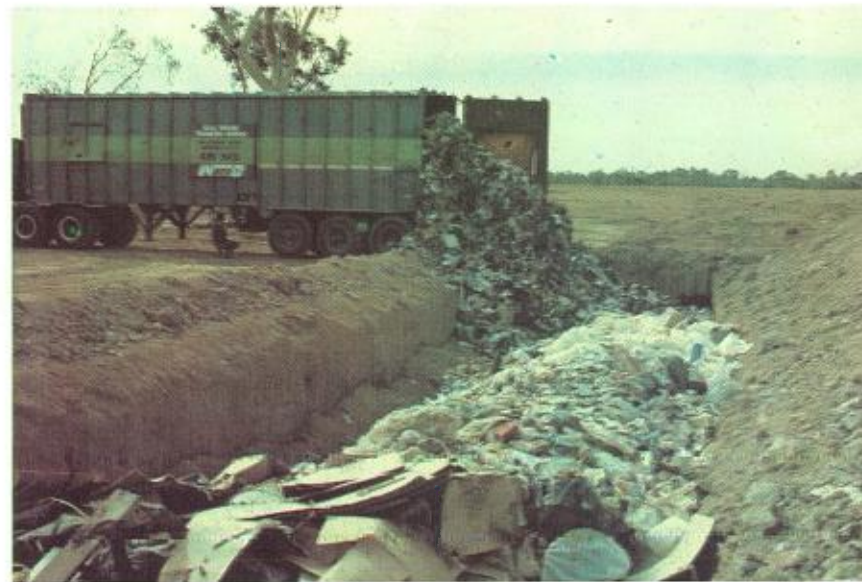
Depositing of dry waste in cell prior to liquid waste receipt
