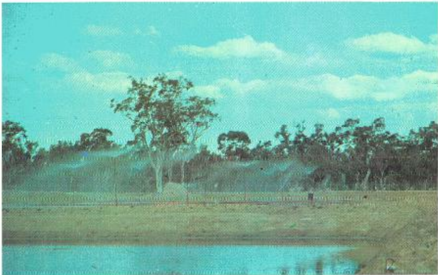
View showing spray evaporation of collected surface waters
