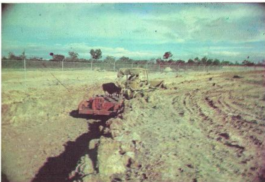
Construction of clay core showing compaction works in progress
