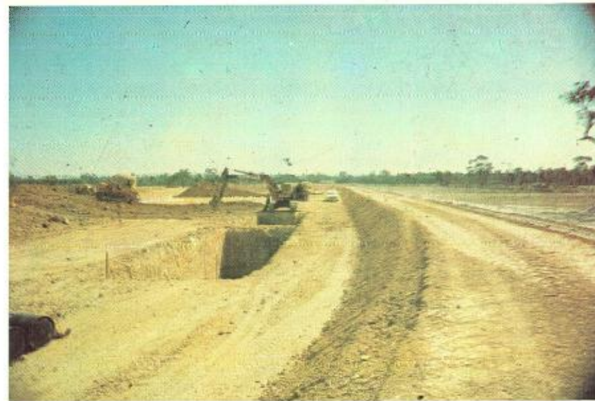
View of bund protection wall and disposal cell construction
